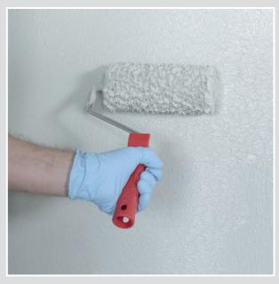
**1** Apply SCHÖNOX iFIX® with the SCHÖNOX iFIX® ROLLER 180 mm in an upright position.
