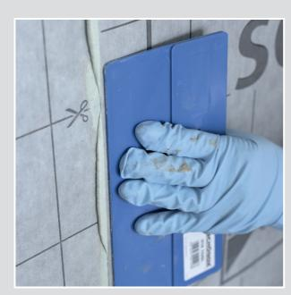
**3** Afterwards press SCHÖNOX AB gently to avoid air bubbles beneath. Remove excess material.
