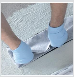
**1** Apply SCHÖNOX iFIX® with the SCHÖNOX ROLLER 100 mm around the floor drain.
