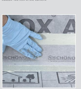
Proceed in the same way with SCHÖNOX ST SEALING TAPE for wall- and wall-/floor connections.
