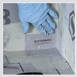
Insert the components like SCHÖNOX ST IC INTERIOR CORNER/SCHÖNOX ST EA EXTERIOR CORNER and avoid air bubbles beneath.
