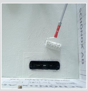
**3** Apply SCHÖNOX iFIX® with the SCHÖNOX ROLLER 180 mm and insert SCHÖNOX AB on the sealing cuff with at least 5 cm overlapping.
