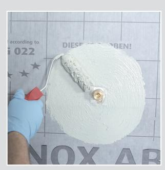
**2** Apply SCHÖNOX iFIX® with the SCHÖNOX ROLLER 100 mm around the plumbing. Insert SCHÖNOX ST DEHNZONENMANSCHETTEN and press it on.
