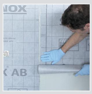
**2** Insert the sheet membrane SCHÖNOX AB into the fresh sealing adhesive (overlapping 5 cm).
