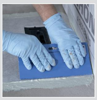
**2** Insert the drain sealing cuff and press it on.
