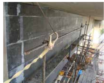
Strengthening with SikaWrap®
