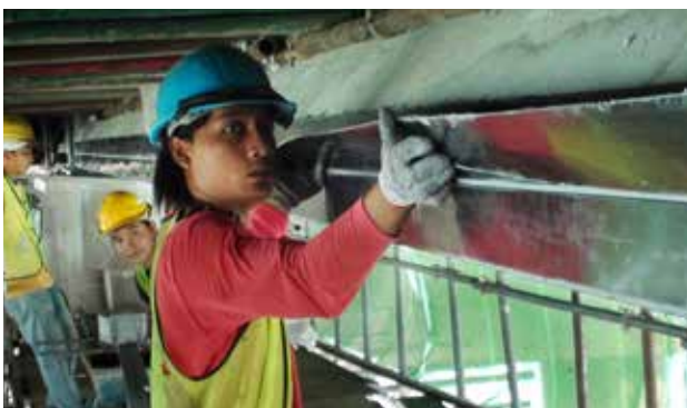
Installation CarboDur®
