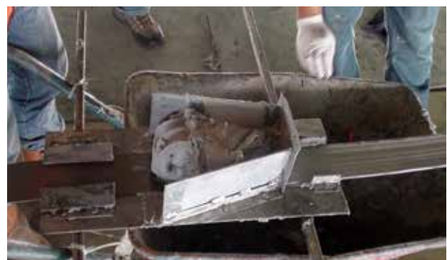
Coating of CarboDur® plates with Sikadur®
