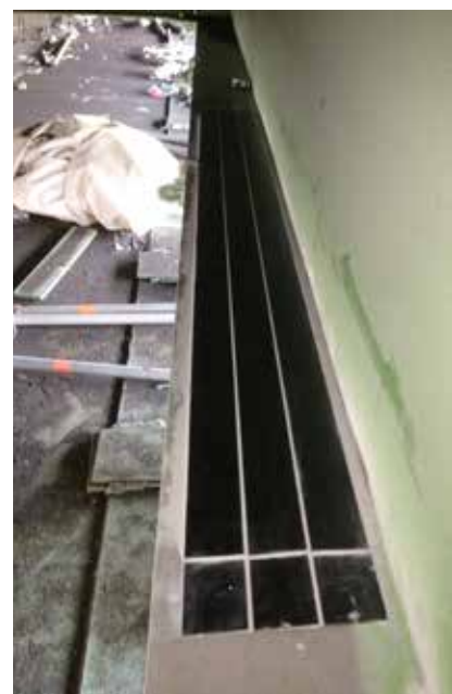
Two layers of Sika CarboDur®
