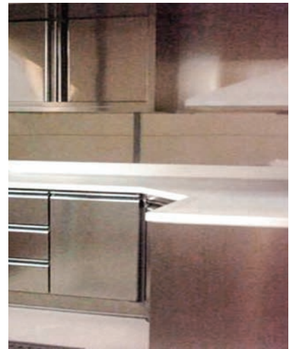
Fig. 8 A galley work surface fitted using Sikaflex®-292i
