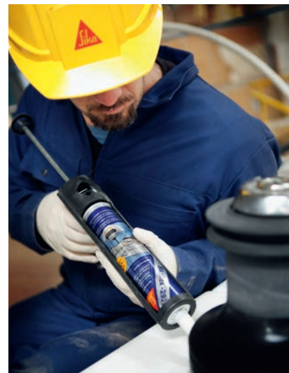
Fig. 2 Applying Sikaflex®-292i
