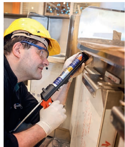
Fig. 9 Application of Sikaflex®-291
