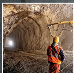
Sprayed concrete
