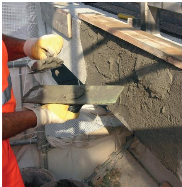
Hand applied mortar
