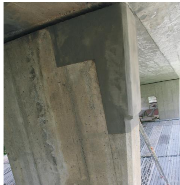
Repair work completed
