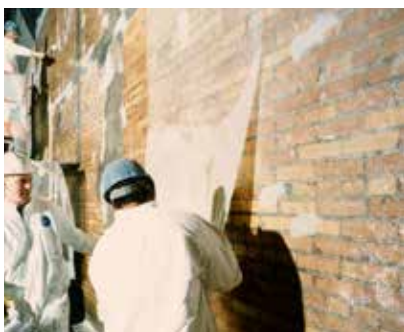
SEISMIC UPGRADING /EARTHQUAKE DAMAGE REPAIR
