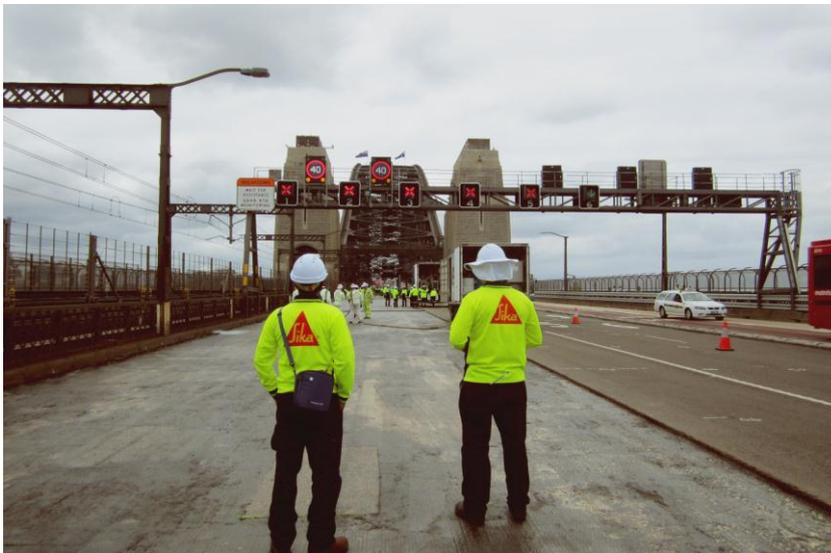
Utilising a fast curing and hard wearing product combination, the Sika waterproofing system was lab tested and trialled over 1000 square metres eight months prior to the final application.
