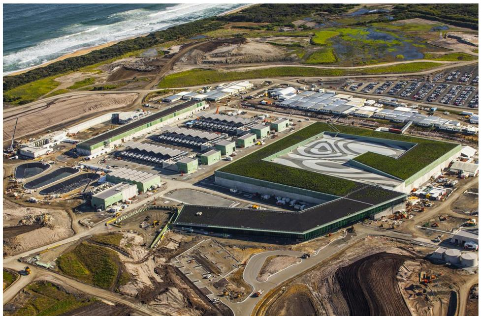
corrosion resistance, thermal control and reduced maintenance, the roof utilises the Sika Sarnafil system which creates a waterproof barrier for the lightweight, structural ply substrate.
