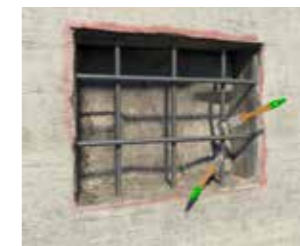
Application of Sika MonoTop®-910 N bonding primer and corrosion protection.
