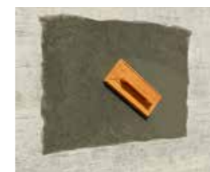
Apply finishing mortar Sika MonoTop®-723 N and smooth the surface using a wooden trowel.
