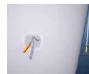
Spreading of resin.
