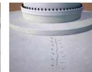
Insert the injection packers.
