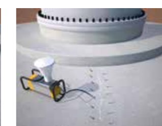
Apply the epoxy resin using a 1-component injection pump.
