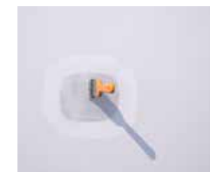
Application of fiber patch and adding Sikadur® Blade Repair Resin.
