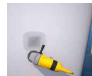
Chamfering of damaged area.
