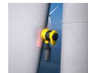
Sanding of repaired area.
