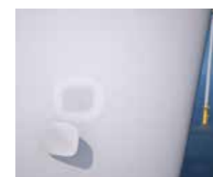
Add fiber patch to build up laminate.
