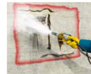
Remove defective concrete and clean the substrate.
