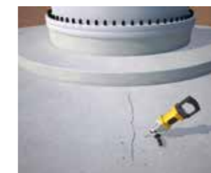
Drill holes for the injection packers.
