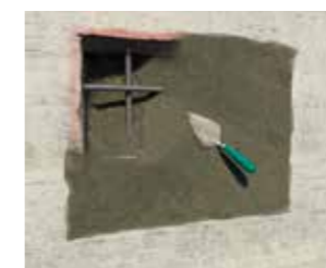
Press Sika MonoTop®-412 N into the repair area using a suitable hand tool.
