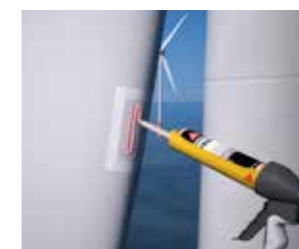
Application of SikaForce®-7800 on prepared surface.
