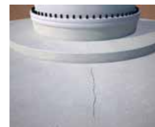
Assess and clean the crack.
