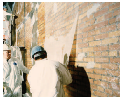
SEISMIC UPGRADING /EARTHQUAKE DAMAGE REPAIR
