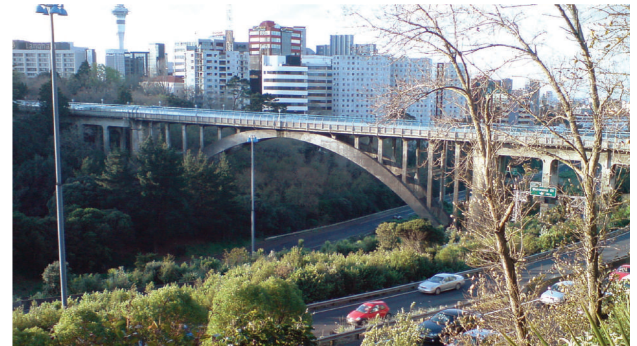
Grafton Bridge, Auckland, New Zealand
