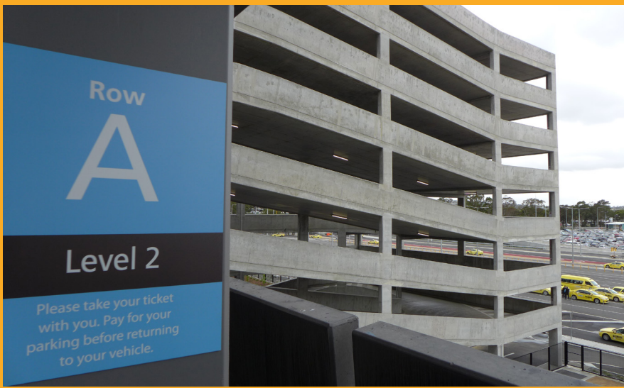
T4 Carpark, Tullamarine Airport, Melbourne
