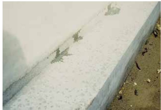
Simple injection process on site
