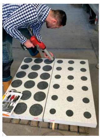
1 After installing the baker rod and applying with Sika<sup>®</sup> Primer-3N for optimal adhesion, the joint is sealed by Sikasil<sup>®</sup>-Pool.
