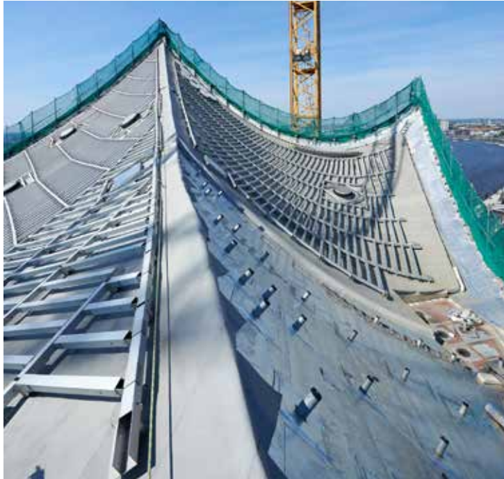
Apart from the Sarnafil® TS 77-20 FPO polymeric membrane, the building also incorporated other products from the Sika Sarnafil system range.
