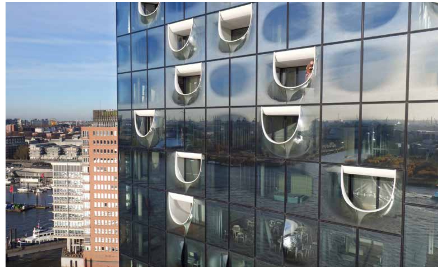
Sika adhesives and sealants were used in the manufacture of the one-off window units for the imposing glass facade.
