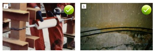
Fig. 8.2: Examples of waterproof joint sealing with swellable adhesive sealants
