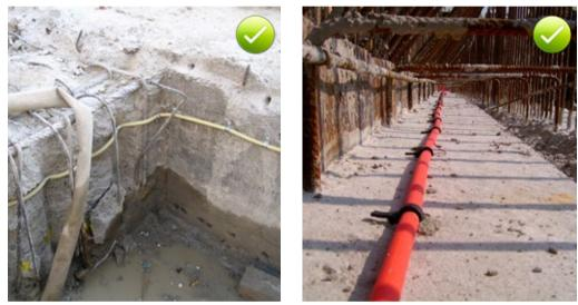
Fig. 9.1: SikaFuko®VT and SikaFuko®ECO injection hose in a construction joint
