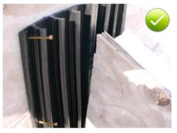
Fig. 5.99: Nailing external waterbars to the wall formwork through their nail strap section
