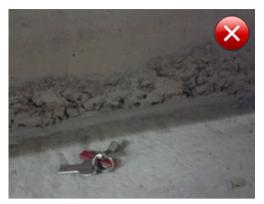
Fig. 2.23: Example of a poor wall base joint with honeycombing
