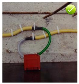
Fig. 9.12: Correct lapping of two injection hose sections
