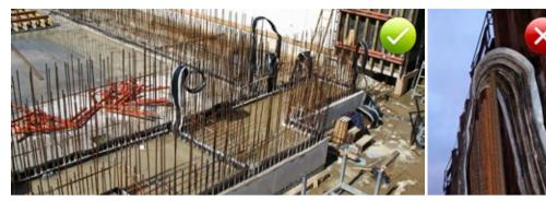
Fig. 5.107: Exposed waterbars in construction joints awaiting the next scheduled pour
