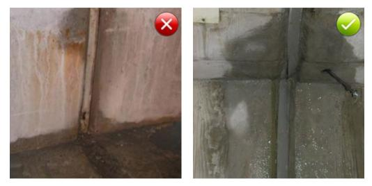
Fig. 15.7: Leaking expansion joint
