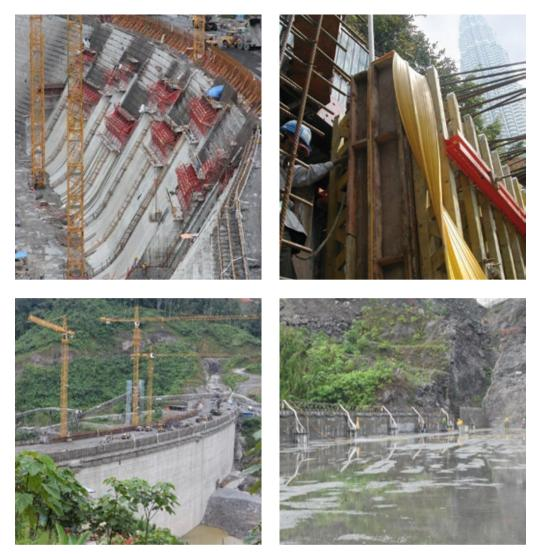
Fig. 5.3: Joint waterproofing with preformed waterbar profiles in dam structures
