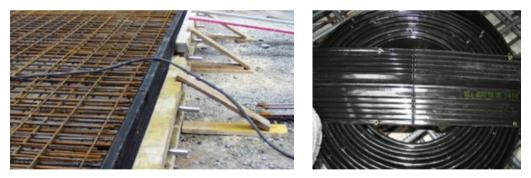
Fig. 5.7: Sika Westec® Waterbars are made from polyethylene (PE) with high chemical resistance
