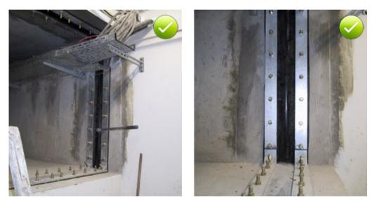
Fig. 15.12: Example of post-sealing of a leaking expansion joint with a clamped waterstop
