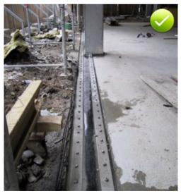
Fig. 13.5: Example of a twin-legged clamped flange system for expansion joint sealing
