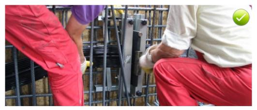
Fig. 14.5: Butt joint welding of Westec® waterbars on site
