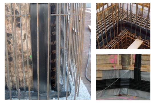
Fig. 5.6: Installing Sika® Tricosal® Tricomer® Waterbars
