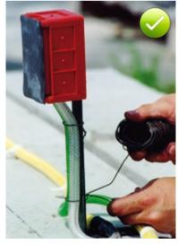
Fig. 9.15: Protective hose end / junction box to safeguard the grouting ends of the installed injection hose system (before formwork erection)
