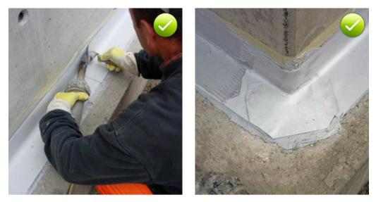
Fig. 10.3: Lap welding of Sikadur-Combiflex® membrane with a hot air welding gun
