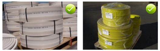
Fig. 5.90: Correct site storage of waterbars on pallets, covered and away from the site access road
