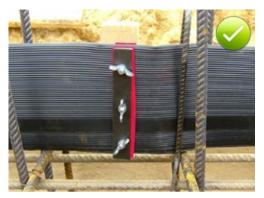
Fig. 7.10: Correct Sika $^{\circ}$  KAB 150 butt joint formation using clamping bars with swellable insert
