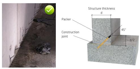
Fig. 15.5: Sealing of a horizontal construction joint by ¬injection grouting through packers
