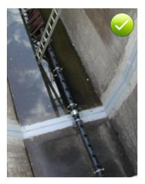
Water side (e.g. swimming pool, sprinkler tank) Specific system adhesive Over-banding, bonded membrane system
