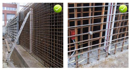
Fig. 12.1: Crack inducing bar with swellable coating for waterproofing the induced joint
