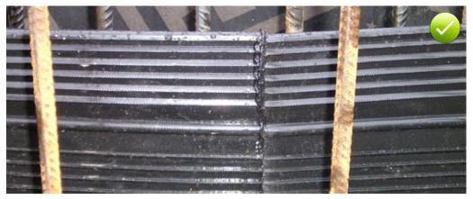
Fig. 14.6: Correctly formed butt joint in a Westec® waterbar
