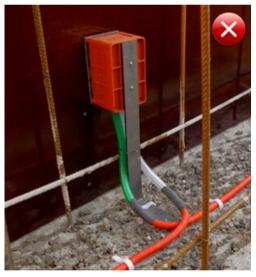
Fig. 9.13: Incorrect lapping of two injection hose sections
