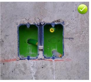
Fig. 9.16: Protective hose end / junction box opened after stripping the wall formwork
