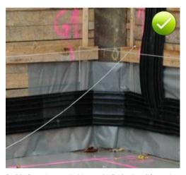
Fig. 5.24: External construction joint waterbar fixed to the wall formwork
