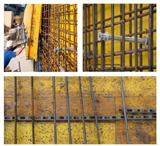
Fig. 2.19: Formwork spacers
