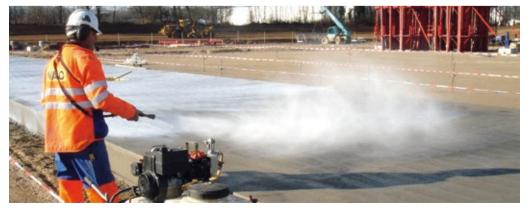
Fig. 2.24: Spray applying liquid curing agent (Sika Antisol®) on the freshly finished concrete surface
