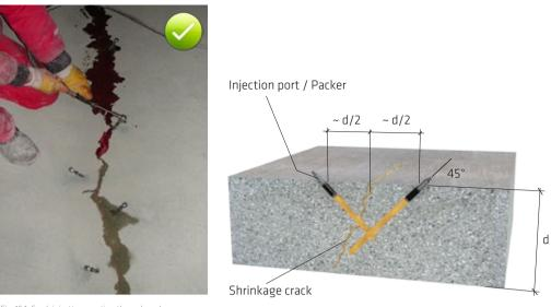
Fig. 15.1: Crack injection grouting through packers
