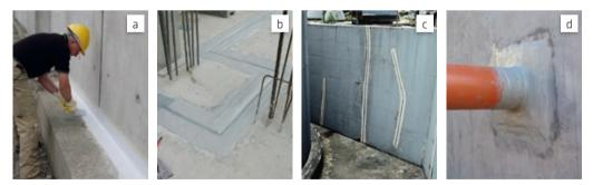
Fig. 10.1: Typical examples of over-banding sealing systems (waterproofing of a: a construction joint, b: an expansion joint, c: cracks, d: a pipe penetration)
