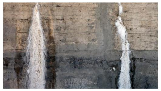
Fig. 2.12: Self-healing of limited sized cracks in concrete
