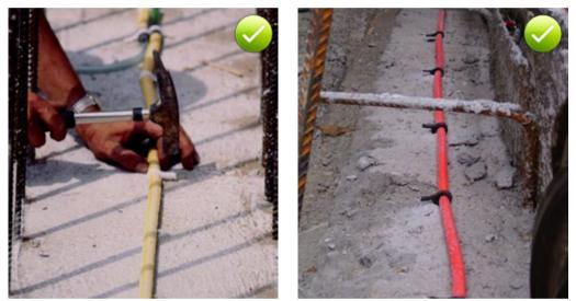
Fig. 9.10: Fixing a SikaFuko® injection hose with special hose clips
