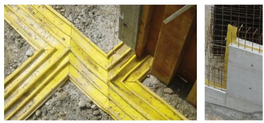
Fig. 5.5: Sika® Waterbars made of PVC-P
