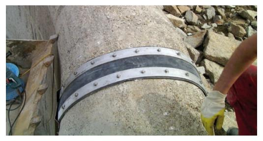
Fig. 5.16b: External clamped waterstop on both sides
