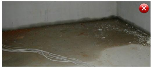
Fig. 15.4: Leaking construction joint(s)
