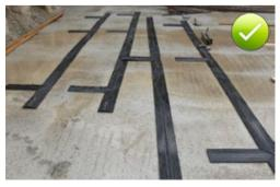
Fig. 5.91: Laying out the waterstop system before installation
