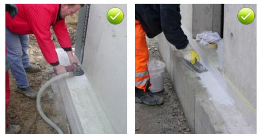
Fig. 10.4: Preparing the substrate
