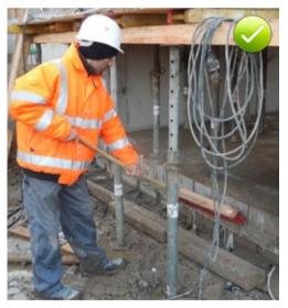
Fig. 5.114: Cleaning the waterbars after the first concreting work
