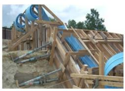
Fig. 5.8: Ethylene vinyl acetate (EVA) waterbars in drinking water installations
