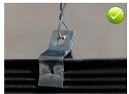
Fig. 5.93: Fixing for internal waterbars
