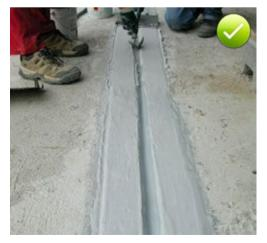
Fig. 10.7: Coating the membrane in the bonded area on both sides of the joint with an additional layer of the epoxy adhesive
