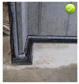
Fig. 13.4: Sealing of an expansion joint between an existing structure and an extension with a single-legged clamped flange system
