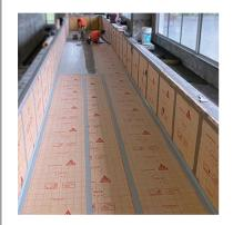
The SCHÖNOX® iFix & AB waterproofing system is a globally proven under tile waterproofing system with un-matched productivity and performance. Unlike typical premixed membranes that are totally reliant of the contractor applying at the correct thickness, SCHÖNOX® iFix & AB system takes away the guess work with a guaranteed film thickness with tiling being able to commence after ½ hour after the application has been installed. Its is also suitable for pools spas and sauna applications.
