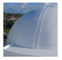
Fast to apply, crack-bridging, polyurethane and polyurea based liquid membranes. Sika liquid applied membranes (LAM) are highly elastic and flexible polymeric systems, usually based on polyurethane or polyurea resins with excellent technical properties for high performance applications. These materials are applied on prepared / primed external concrete surfaces by spraying and provide excellent solutions for complex detailing.
