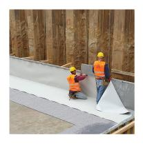
SikaProof<sup>®</sup> A+ is the second generation of Sika's fully adhered membrane systems. The innovative feature of a "one tape application" and the option to thermally joint the laps, makes it an obvious choice for any good installer. The benefits of the SikaProof<sup>®</sup> A+ have proven to have a 30% faster application time than the conventional system.
