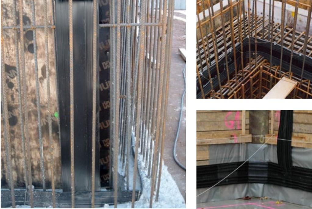
Fig. 5.6: Installing Sika® Tricosal® Tricomer® Waterbars
