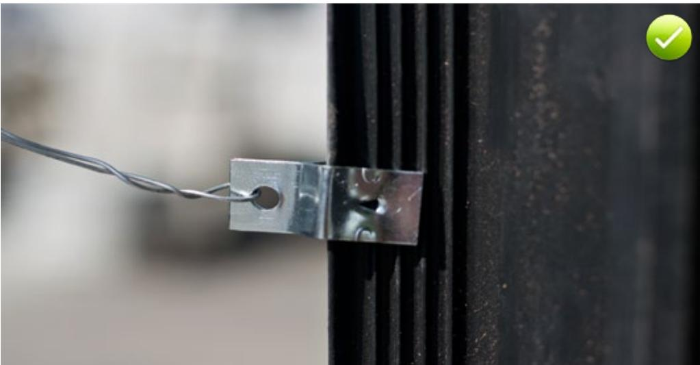
Fig. 11.4: Fixing the crack inducing sealing tube with waterstop clips
