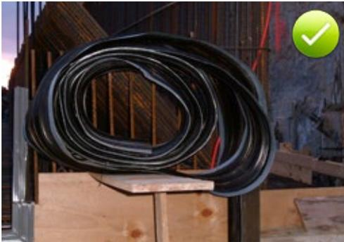
Fig. 5.109: Correct care and protection of the waterbars until the next section is concreted
