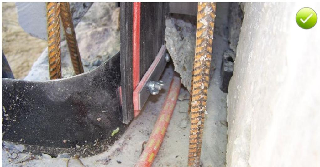
Fig 7.11: Connection of a Sika® KAB 125 combined construction joint waterbar to a thermo-plastic expansion joint waterbar by clamping bars with swellable insert
