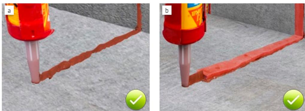
Fig. 8.8: Fixing a swellable profile by adhesive bonding (a: applying the adhesive sealant, b: pressing the profile into the fresh adhesive sealant)
