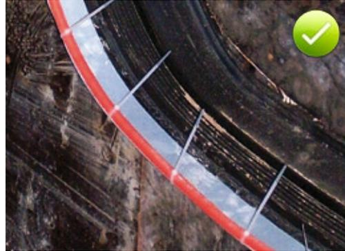
Fig. 9.5: Injection hose fixed on the Sika® Tricosal® FMS waterbar with plastic ties (to be cut)
