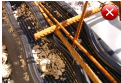
Fig. 5.106: Stop end rib anchors deformed by placing the reinforcement too close and directly on top in fact
