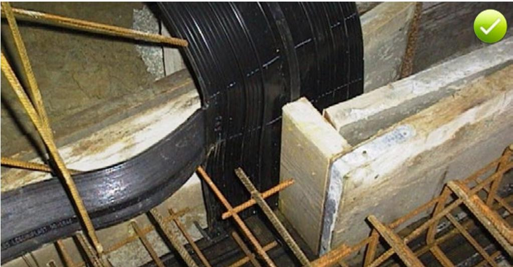
Fig. 7.8: Connection of a KAB combined construction joint waterbar to a thermo-plastic expansion joint waterstop by heat welding
