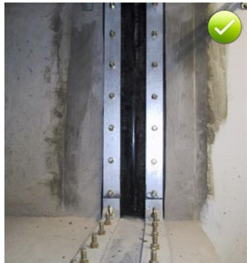
Fig. 15.12: Example of post-sealing of a leaking expansion joint with a clamped waterstop
