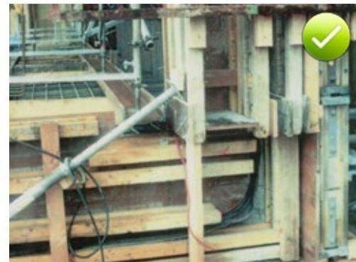
Fig. 5.103: Waterbar stop end formwork to the base slab
