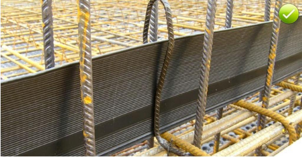
Fig. 7.5: Special rhombic clips to fix the Sika® KAB 150 combined waterstop system
