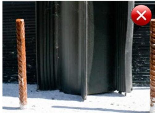
Fig. 11.7: Base of an incorrectly installed crack inducing sealing tube with insufficient clearance from the construction joint
