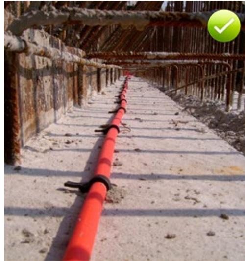
Fig. 9.1: SikaFuko®VT and SikaFuko®ECO injection hose in a construction joint
