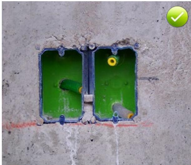
Fig. 9.16: Protective hose end / junction box opened after stripping the wall formwork
