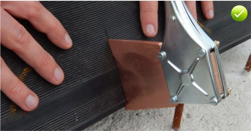
Fig. 7.7: Forming a butt joint by thermoplastic welding with a welding axe
