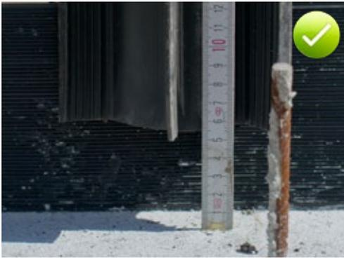
Fig. 11.6: Base of a correctly installed crack inducing sealing tube
