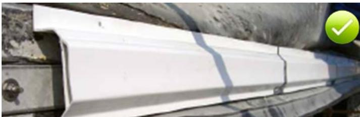
Fig. 13.9: Clamped joint protected against shearing off under stress by a special clamp protection profile with a movement void
