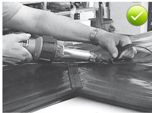
Fig. 5.80: Reinforcing the weld during prefabrication of the waterbar by using a hot air gun to weld on a reinforcing strip of the same material
