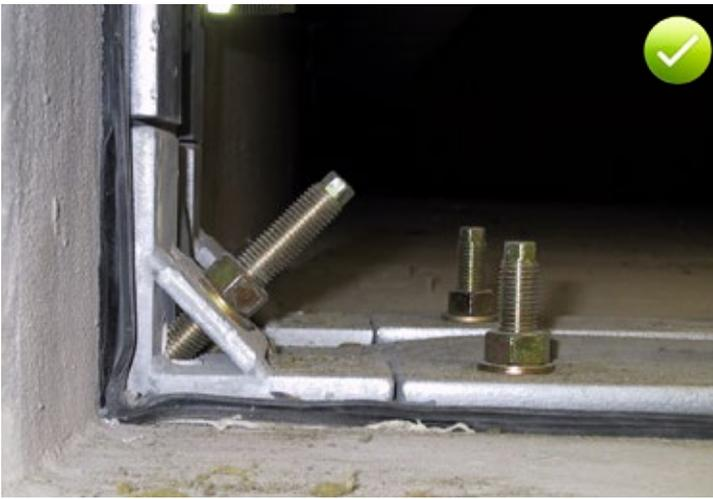
Fig. 13.7: Example of correct formation of an internal corner with a non-standard clamped flange
