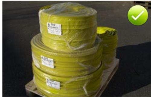
Fig. 5.90: Correct site storage of waterbars on pallets, covered and away from the site access road
