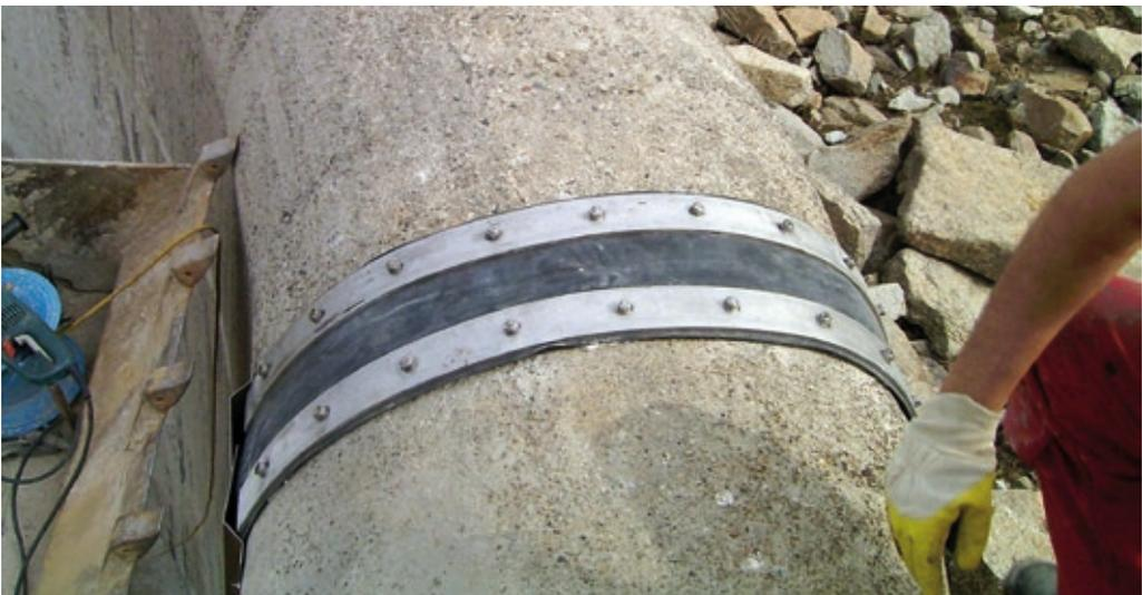
Fig. 5.16b: External clamped waterstop on both sides
