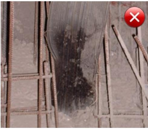
Fig. 5.28: Internal construction joint waterbar with inadequate clearance from the starter bars
