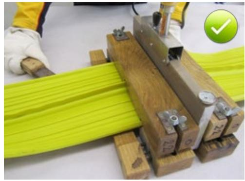
Fig. 5.67: Melting the waterbar ends by pressing them both against the hot welding blade with the lever closing mechanism
