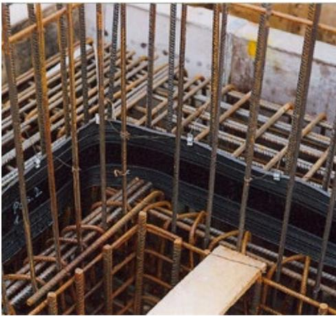
Fig. 5.21: Construction joint waterbar with top reinforcement break
