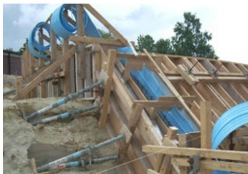
Fig. 5.8: Ethylene vinyl acetate (EVA) waterbars in drinking water installations
