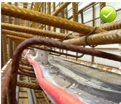
Fig. 5.26: Waterstop system with the correct clearance from the reinforcement
