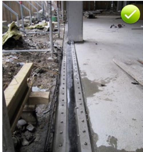
Fig. 13.5: Example of a twin-legged clamped flange system for expansion joint sealing
