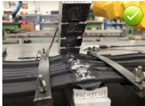
Fig. 5.89: Butt joint after vulcanisation
