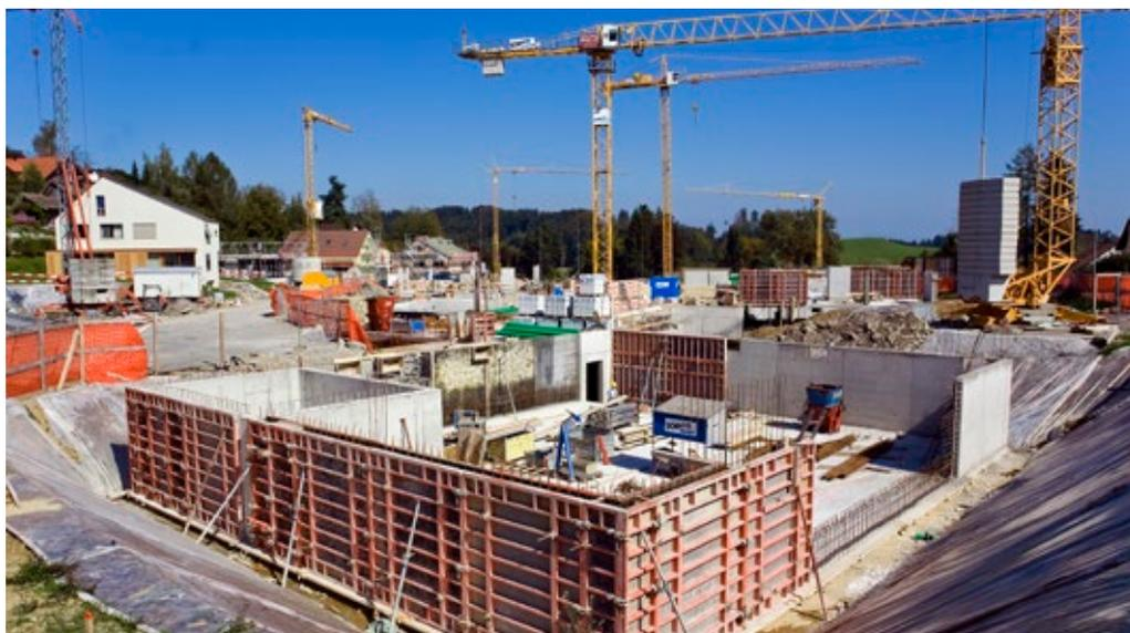
Fig. 2.3: Example of a relatively simple, rectangular, single-storey basement built to be durably watertight with a Sika Watertight Concrete System
