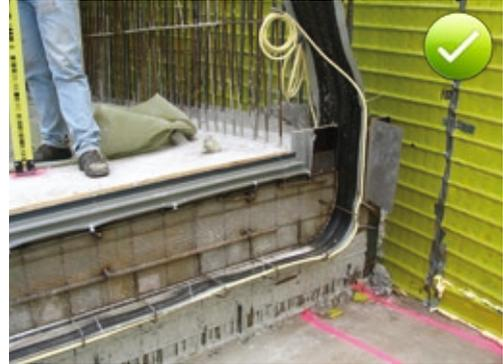
Fig. 5.96: Correct concrete cover to the first anchor rib of  $\geq 30$  mm (approx. 1 1/8") for an internal expansion joint waterbar in the first concrete section
