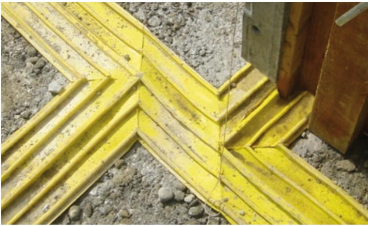
Fig. 5.61: Example of a prefabricated section of a waterbar waterstopping system
