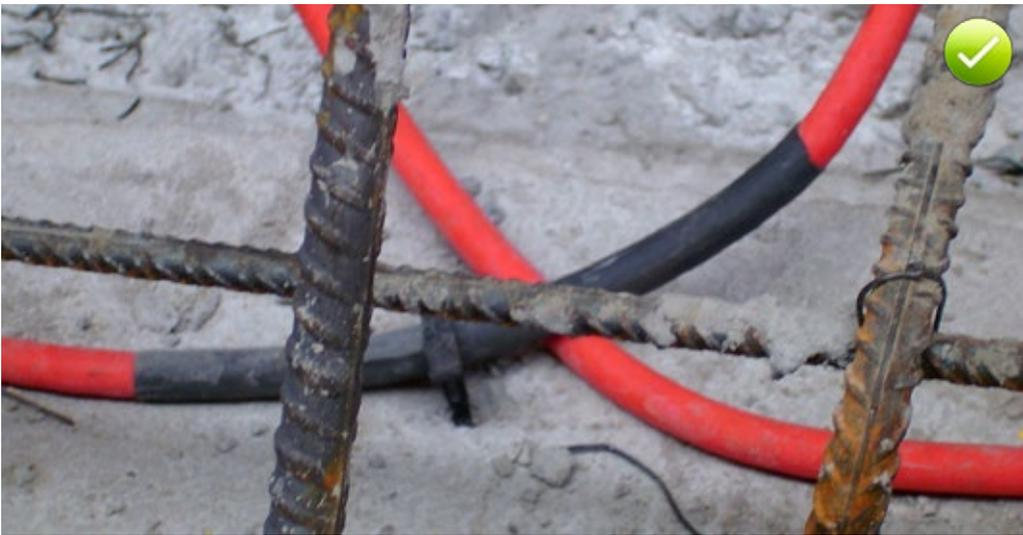
Fig. 9.11: Correctly formed overlap jointing of two injection hoses
