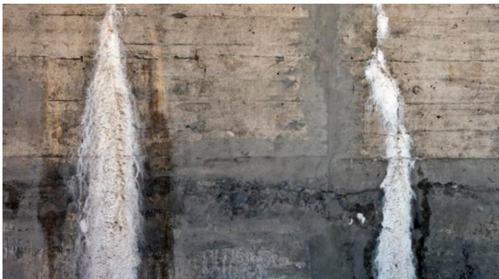
Fig. 2.12: Self-healing of limited sized cracks in concrete
