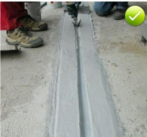
Fig. 10.7: Coating the membrane in the bonded area on both sides of the joint with an additional layer of the epoxy adhesive
