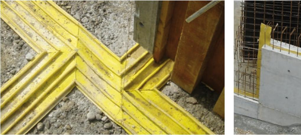
Fig. 5.5: Sika® Waterbars made of PVC-P
