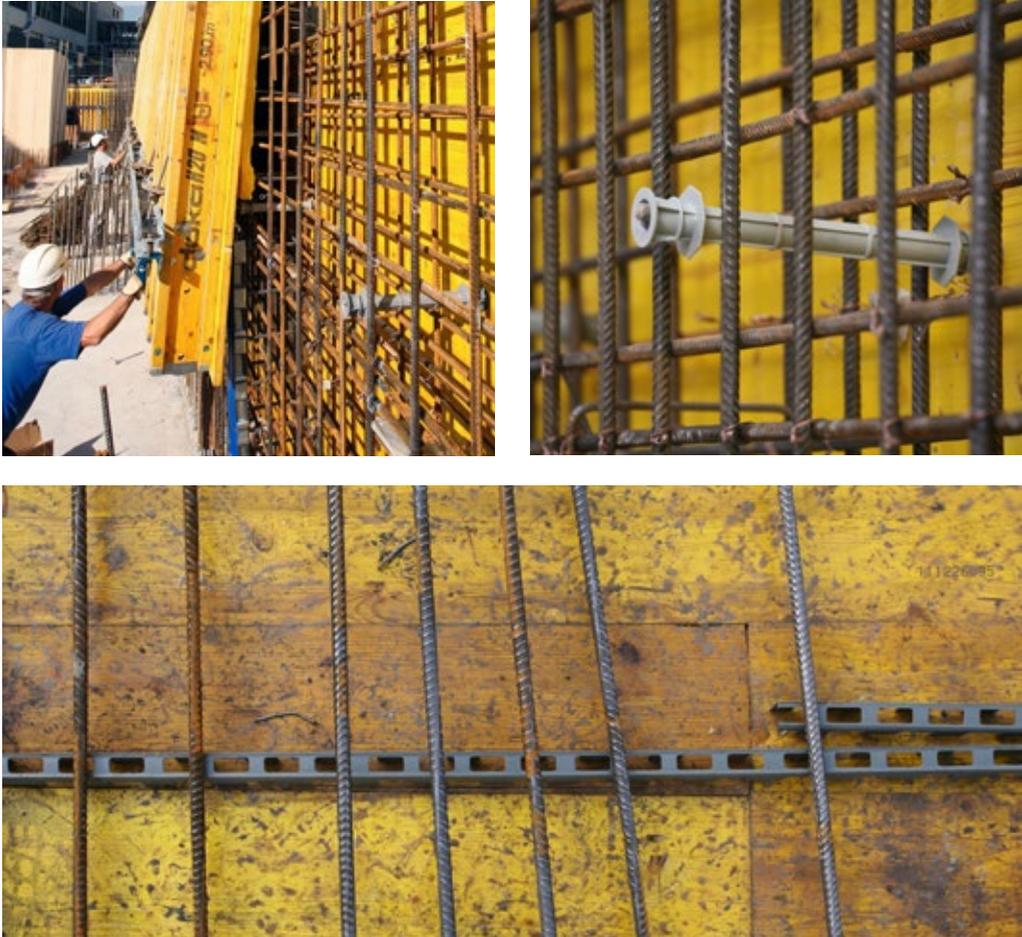
Fig. 2.19: Formwork spacers
