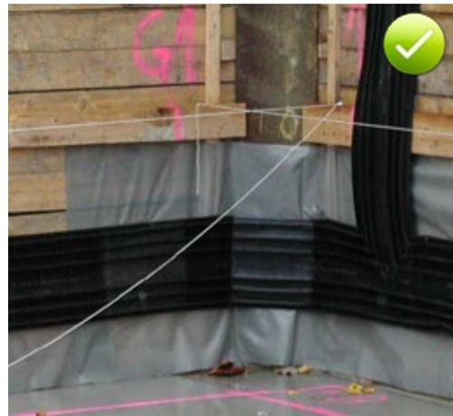
Fig. 5.24: External construction joint waterbar fixed to the wall formwork
