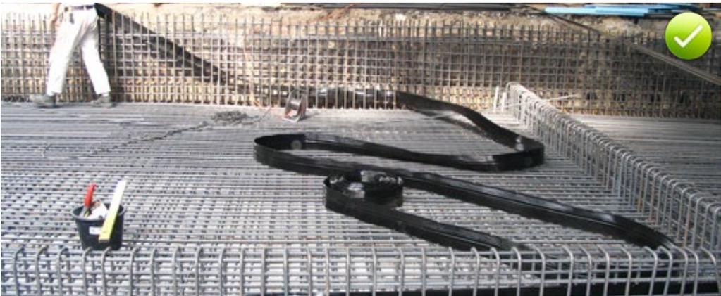
Fig. 14.7: Westec® waterbar installed in a kicker to be poured with the base slab
