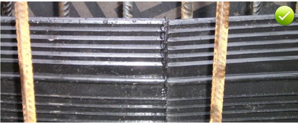
Fig. 14.6: Correctly formed butt joint in a Westec® waterbar
