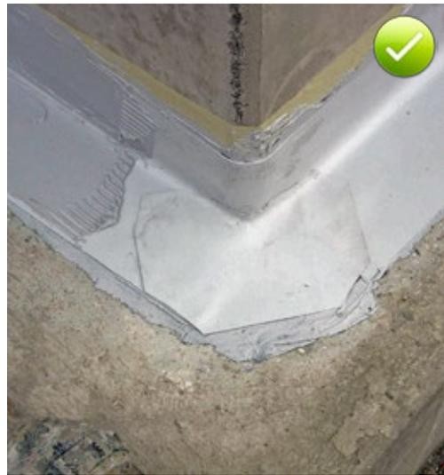
Fig. 10.3: Lap welding of Sikadur-Combiflex® membrane with a hot air welding gun
