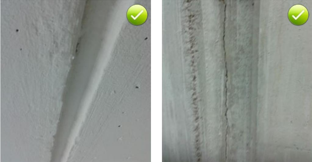
Fig. 11.3: Groove for crack formation in an induced crack section
