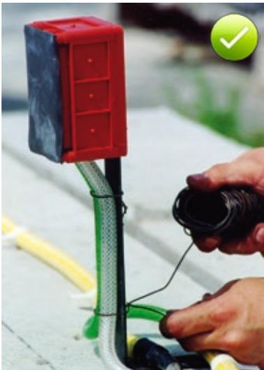
Fig. 9.15: Protective hose end / junction box to safeguard the grouting ends of the installed injection hose system (before formwork erection)
