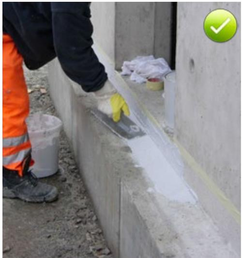
Fig. 10.4: Preparing the substrate
