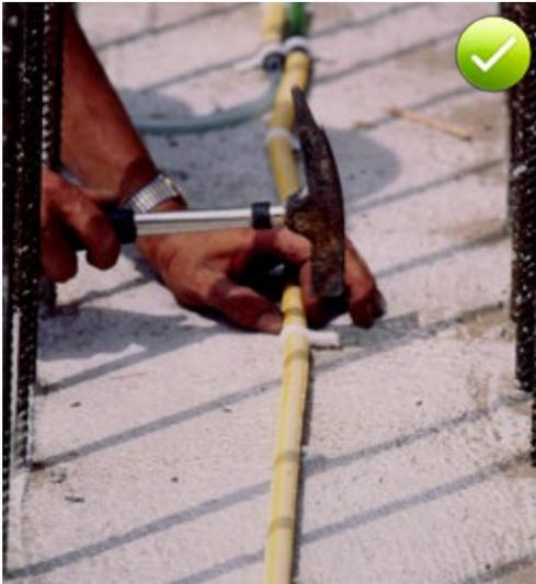
Fig. 9.10: Fixing a SikaFuko® injection hose with special hose clips
