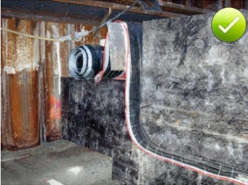
Fig. 9.4: Stop-end formwork for a base slab with an Sika® Tricosal® FMS waterbar and additional injection hose for secondary waterproofing
