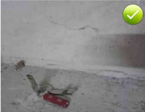
Fig. 2.22: Wall with a correctly concreted base layer
