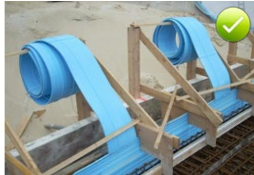
Fig. 5.110: Correct care and protection of the waterbar until the next section is concreted
