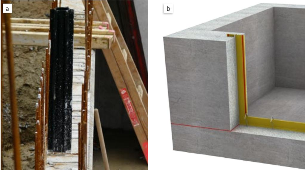
Fig. 4.3: Crack inducers for forming controlled crack induced joints (a: controlled crack sealing tube, b: KAB 175 SR)
