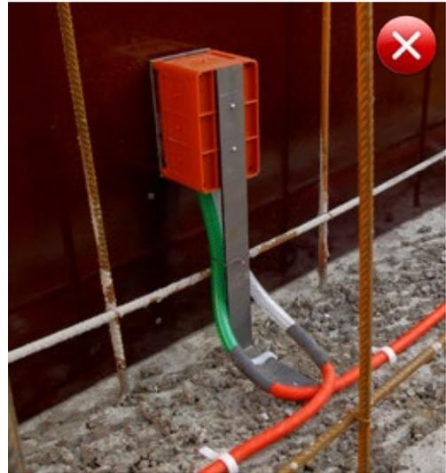
Fig. 9.13: Incorrect lapping of two injection hose sections
