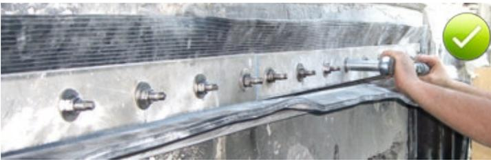
Fig. 13.8: Retightening the clamp to the specified tightening torque
