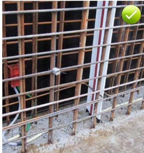
Fig. 12.1: Crack inducing bar with swellable coating for waterproofing the induced joint
