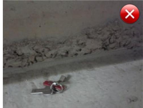
Fig. 2.23: Example of a poor wall base joint with honeycombing
