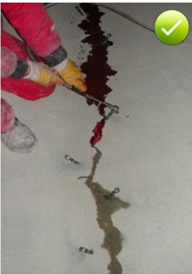
Fig. 15.1: Crack injection grouting through packers
