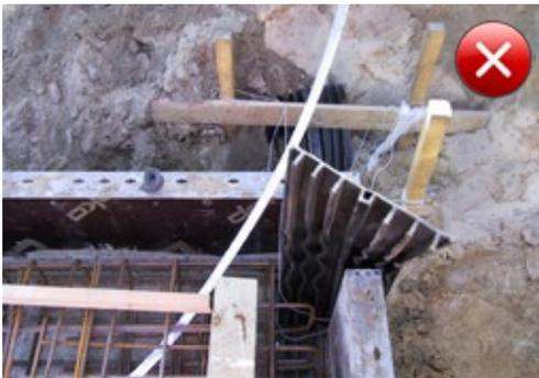
Fig. 5.35: Poor example showing a free connecting end of an external waterbar which is too short
