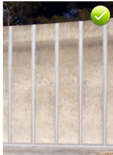
Fig. 15.3: Sealing cracks by over-banding with the Sikadur-Combiflex®SG system
