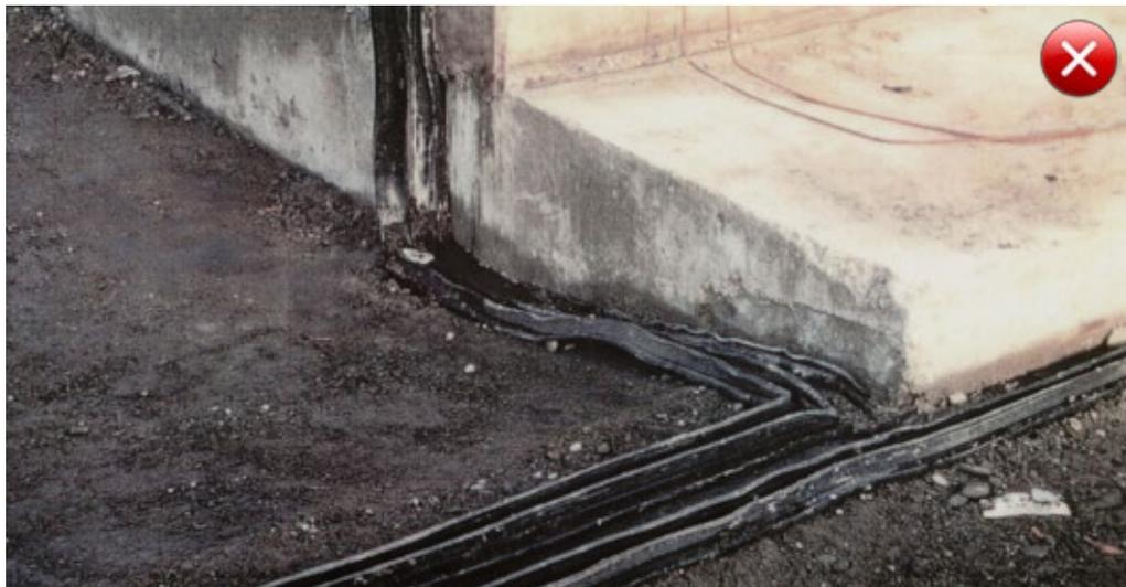
Fig. 5.112: Dirty and contaminated waterbars after concreting the first section of a base slab, now requiring thorough cleaning and inspection before concreting
