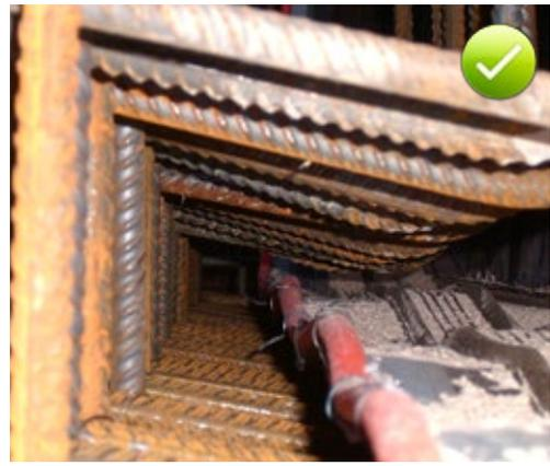
Fig. 5.29: Correctly installed internal construction joint waterbar with sufficient clearance from the starter bars
