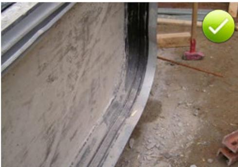
Fig. 5.111: Properly cleaned external waterbar to be cast in a floor slab
