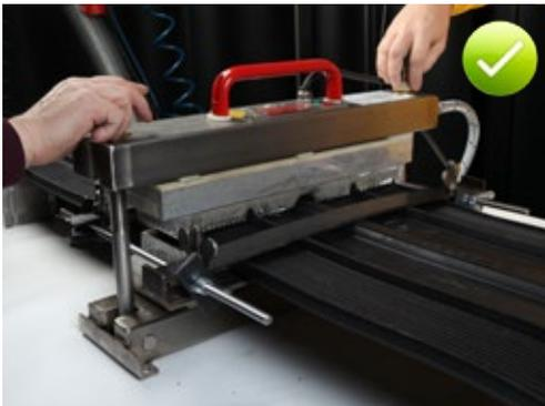
Fig. 5.88: Forming a butt joint in an elastomer waterbar with a vulcanizer
