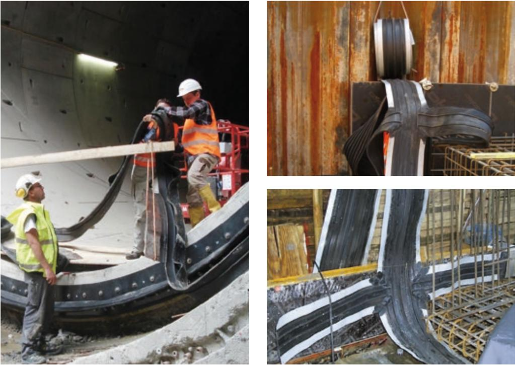
Fig. 5.9: Typical Sika® Tricosal® elastomer waterbars installations
