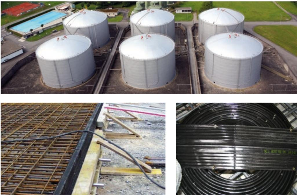
Fig. 5.7: Sika Westec® Waterbars are made from polyethylene (PE) with high chemical resistance
