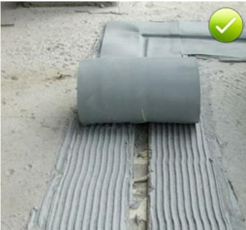
Fig. 10.5: Rolling out the membrane into the adhesive bed
