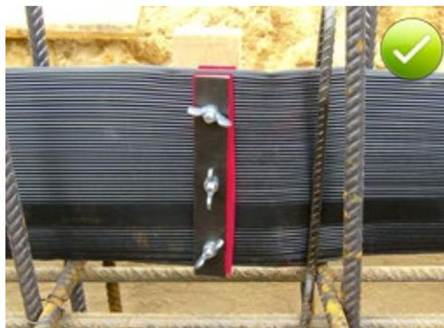
Fig. 7.10: Correct Sika® KAB 150 butt joint formation using clamping bars with swellable insert
