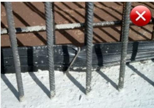
Fig. 5.105: Waterbar damaged and folded over by pedestrian traffic that must clearly be prevented
