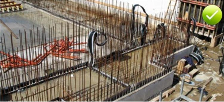
Fig. 5.107: Exposed waterbars in construction joints awaiting the next scheduled pour
