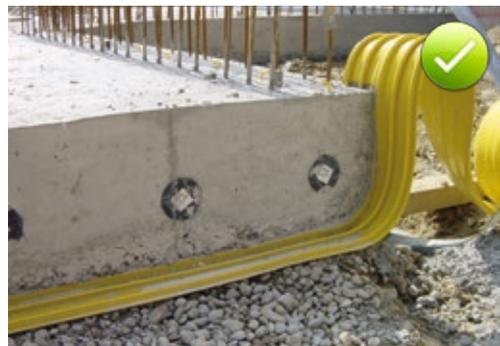
Fig. 5.36: External waterbar in the base slab with change of direction in minimum bending radius
