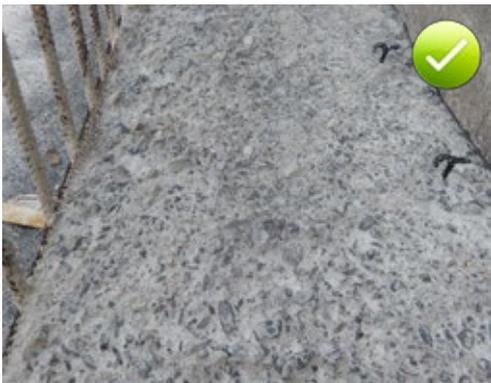
Fig. 3.8: Construction joints properly prepared and cleaned of cement laitance
