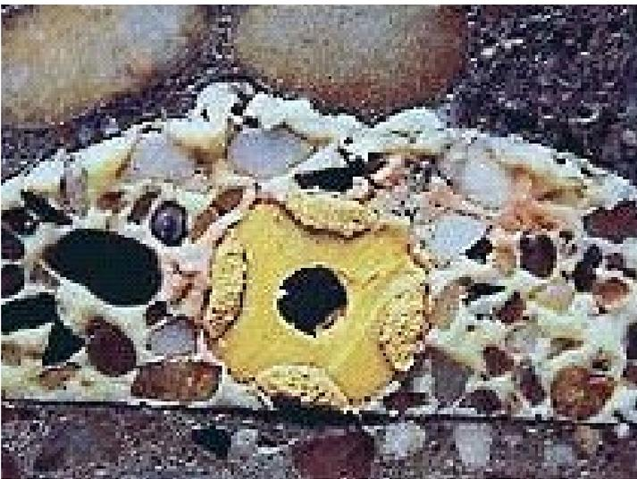
Fig. 9.2: Honeycombing grouted and sealed with an acrylate resin through a SikaFuko®VT-1 injection hose
