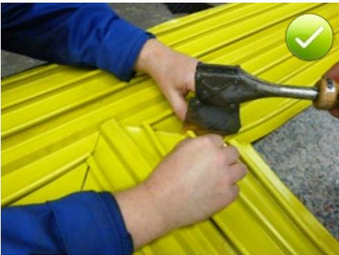
Fig. 5.77: Prefabrication of a flat T-piece for an external thermoplastic waterbar with a welding axe
