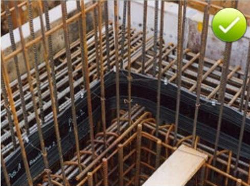
Fig. 5.92: Waterbars installed in the construction joint between base slab and wall with continuous top reinforcement layer
