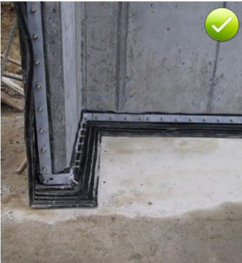
Fig. 13.4: Sealing of an expansion joint between an existing structure and an extension with a single-legged clamped flange system
