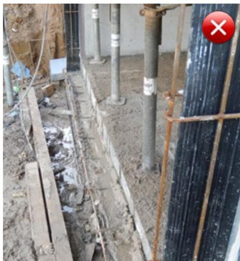
Fig. 5.113: Dirty and contaminated waterbars after concreting the first section of a base slab, now requiring thorough cleaning and inspection before concreting
