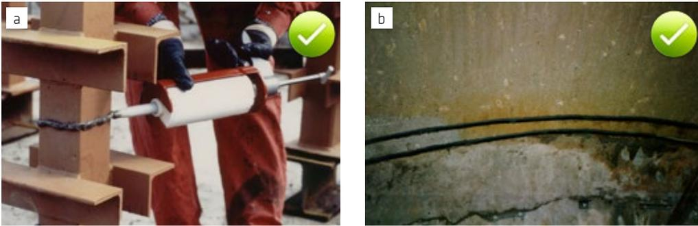
Fig. 8.2: Examples of waterproof joint sealing with swellable adhesive sealants
