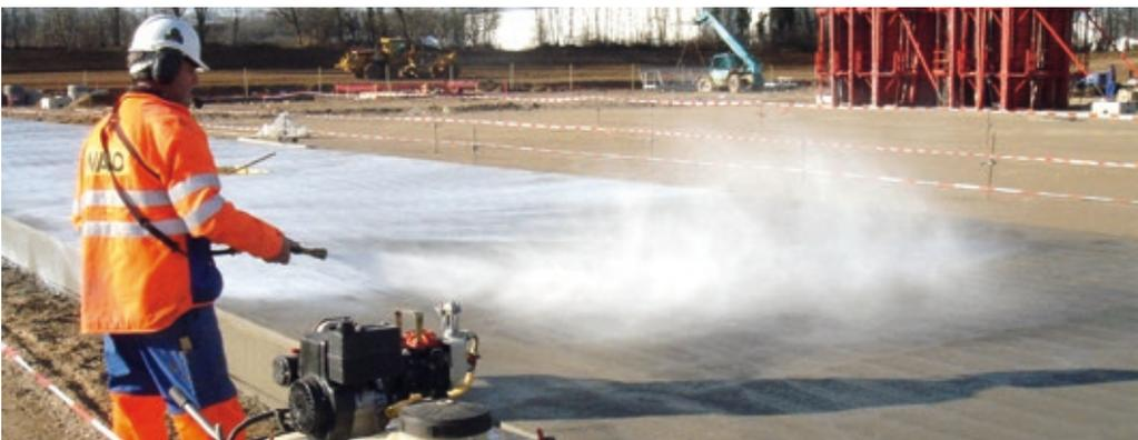
Fig. 2.24: Spray applying liquid curing agent (Sika Antisol®) on the freshly finished concrete surface
