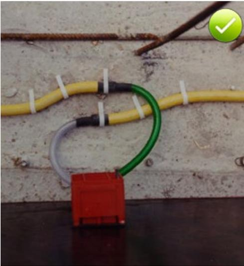
Fig. 9.12: Correct lapping of two injection hose sections
