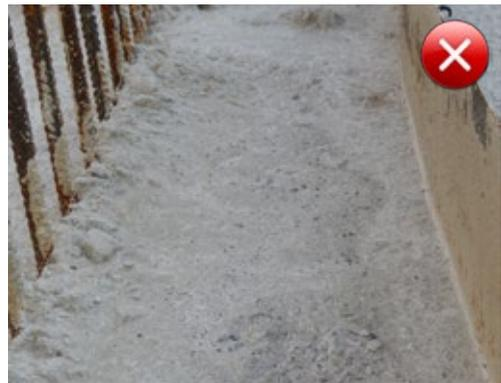
Fig. 3.9: Close up of a construction joint surface with heavy cement laitance
