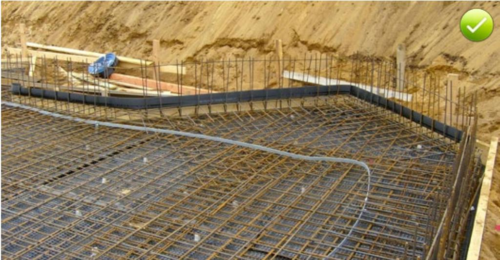
Fig. 7.4: Sika® KAB 150 on the top reinforcement layer before the base slab is concreted
