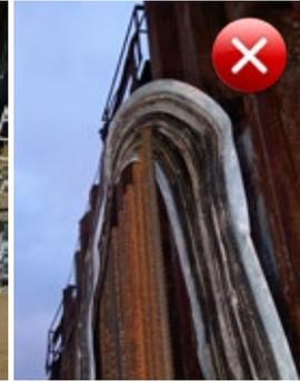
Fig. 5.108: Damage caused to the waterbar by it not being properly protected
