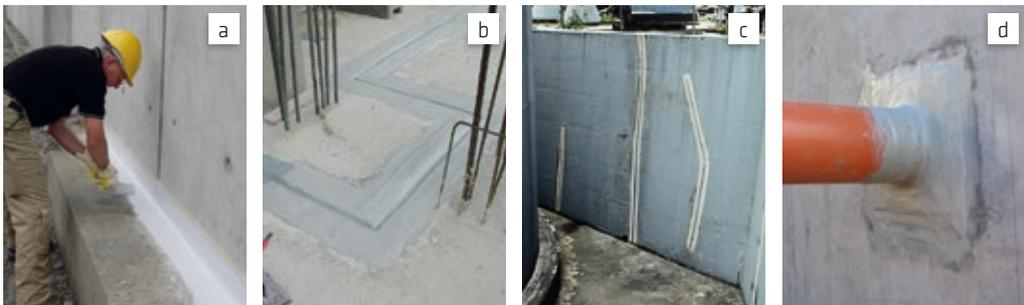
Fig. 10.1: Typical examples of over-banding sealing systems (waterproofing of a: a construction joint, b: an expansion joint, c: cracks, d: a pipe penetration)
