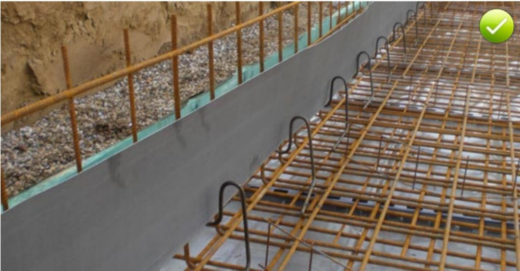
Fig. 6.1: Metal waterbar in a construction joint between a base slab and wall
