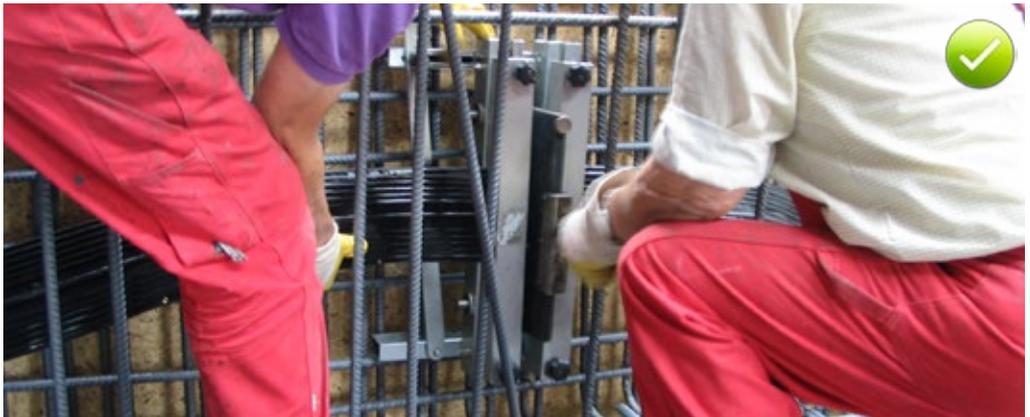
Fig. 14.5: Butt joint welding of Westec® waterbars on site
