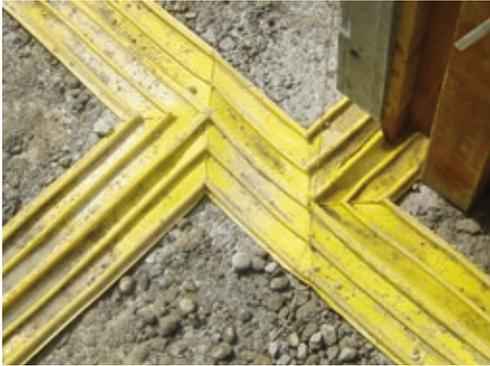
Fig. 5.97: External movement joint waterbar waterstopping system installed on the concrete blinding layer
