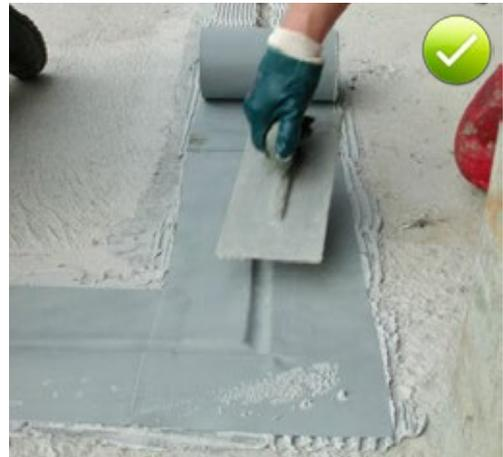
Fig. 10.6: Pressing the membrane into the adhesive bed
