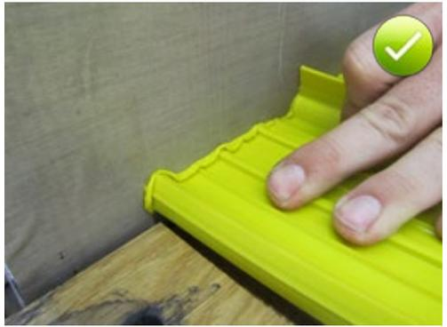
Fig. 5.69: Melting process at the waterbar end in contact with the hot welding blade
