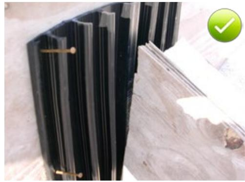
Fig. 5.100: Fixing an external expansion joint waterbar to the nail strap with nails after the first half has been concreted in
