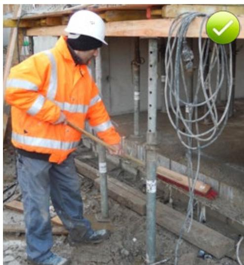
Fig. 5.114: Cleaning the waterbars after the first concreting work
