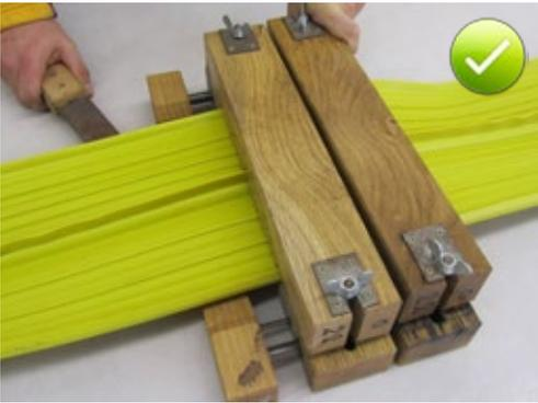
Fig. 5.68: Pressing the two molten waterbar ends together with the lever closing mechanism of the jig after removing the welding blade
