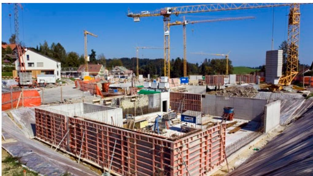
Fig. 2.3: Example of a relatively simple, rectangular, single-storey basement built to be durably watertight with a Sika Watertight Concrete System
