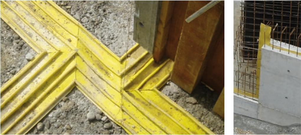
Fig. 5.5: Sika® Waterbars made of PVC-P
