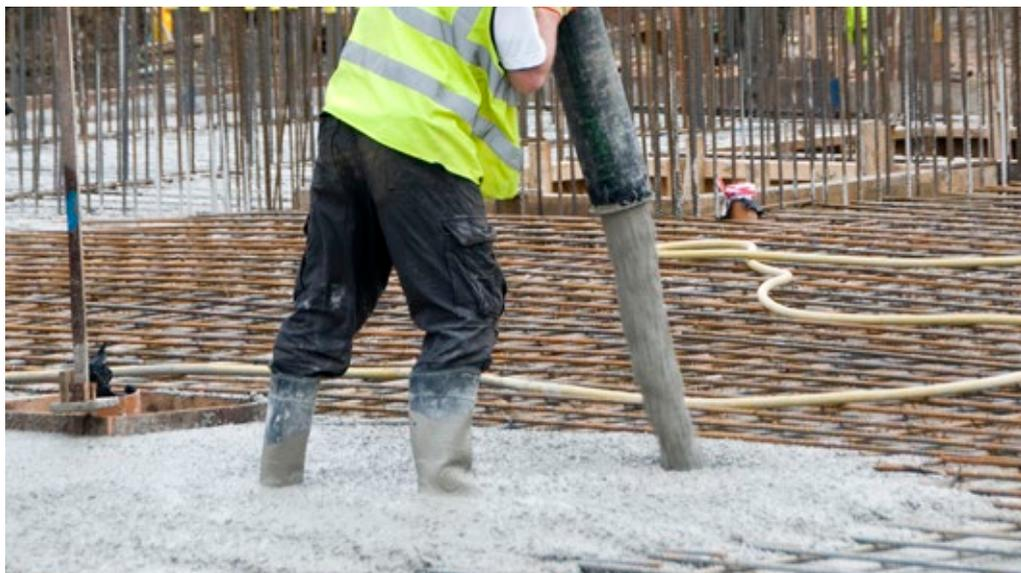
Fig. 2.2: Concreting with an easily placed and compacted Sika Waterproof Concrete
