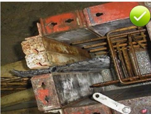
Fig. 5.102: Waterbar stop end formwork for a wall
