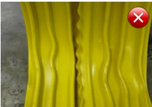
Fig. 5.37: Warping of anchor ribs on an external waterbar with high anchoring ribs installed in the radius
