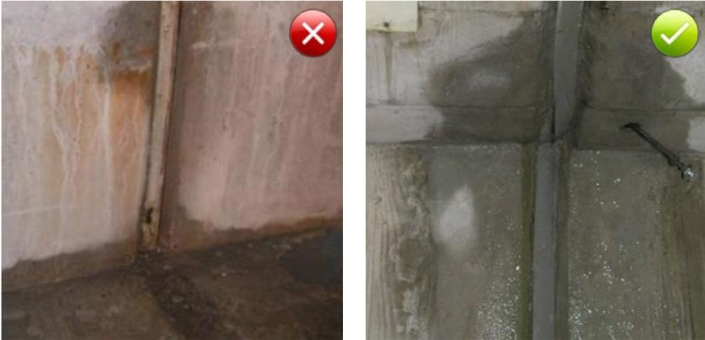
Fig. 15.7: Leaking expansion joint
