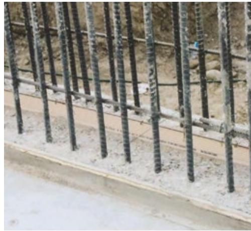
Fig. 5.22: Construction joint waterbar with concrete kicker
