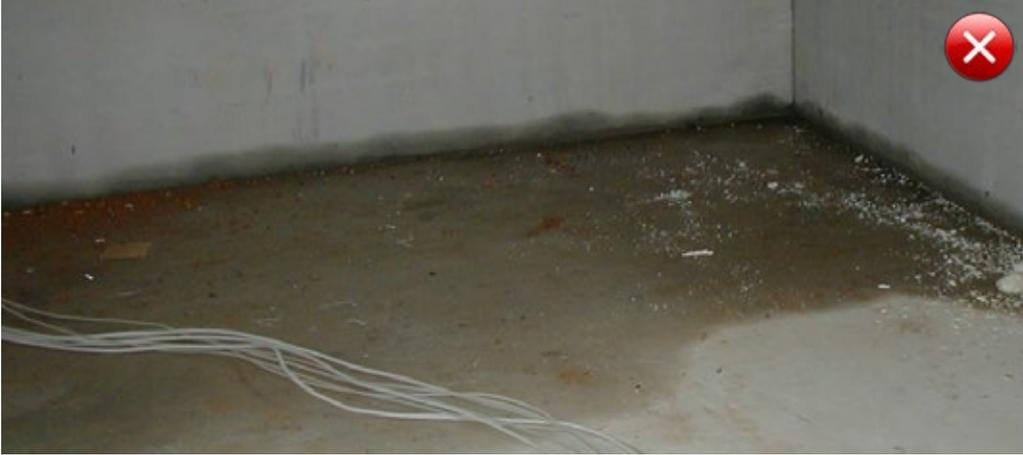
Fig. 15.4: Leaking construction joint(s)
