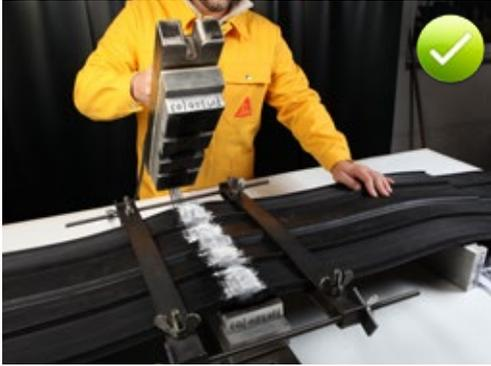
Fig. 5.86: Placing the waterbar with the prepared butt joint in the vulcanizer
