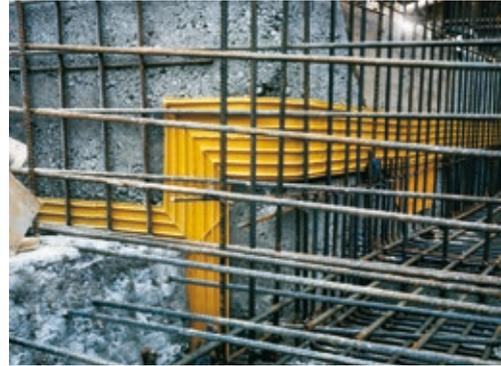
Fig. 5.98: External construction joint waterbar fixed on an existing adjacent wall
