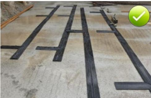
Fig. 5.91: Laying out the waterstop system before installation
