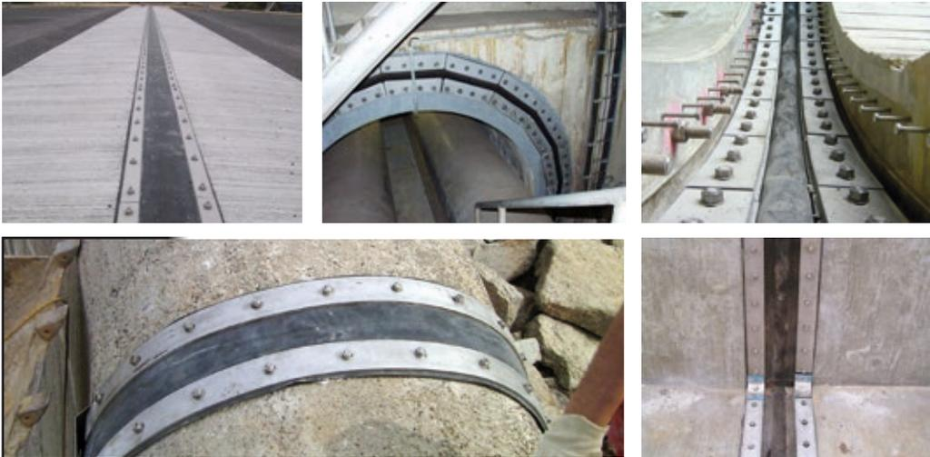
Fig. 13.1: Typical applications of clamped flange expansion joint sealing solutions
