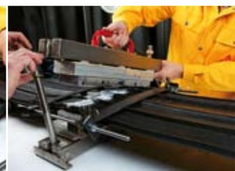
Powdering of waterstop and inserting into the vulcanizing equipment
