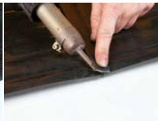
Strengthening with welding foil using hot air gun
