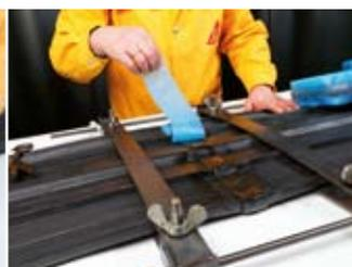
Joining the waterstop, tightening with the fixing Clamps
