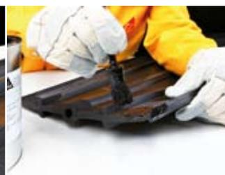
Applying the vulcanizing solution to the rubber surface
