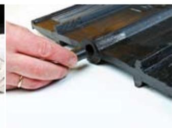
Plugging of the centre bulb with a cellular foam plug and inserting a raw rubber plug
